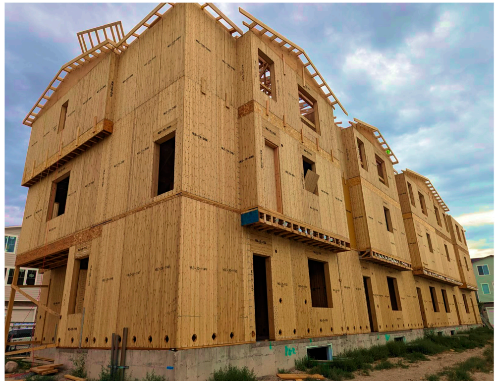
Figure 5. International Building Code-compliant multifamily building in Salt Lake City, UT, USA. Six-unit town home buildings, each unit average size 160+ sq meters, one of six similar multifamily buildings. As shown, the building is 3 stories on concrete slab with envelope framed from low-embodied carbon, high-thermal efficiency, off-site pre-fabricated bamboo–wood composite vertical framing (wall) system.
