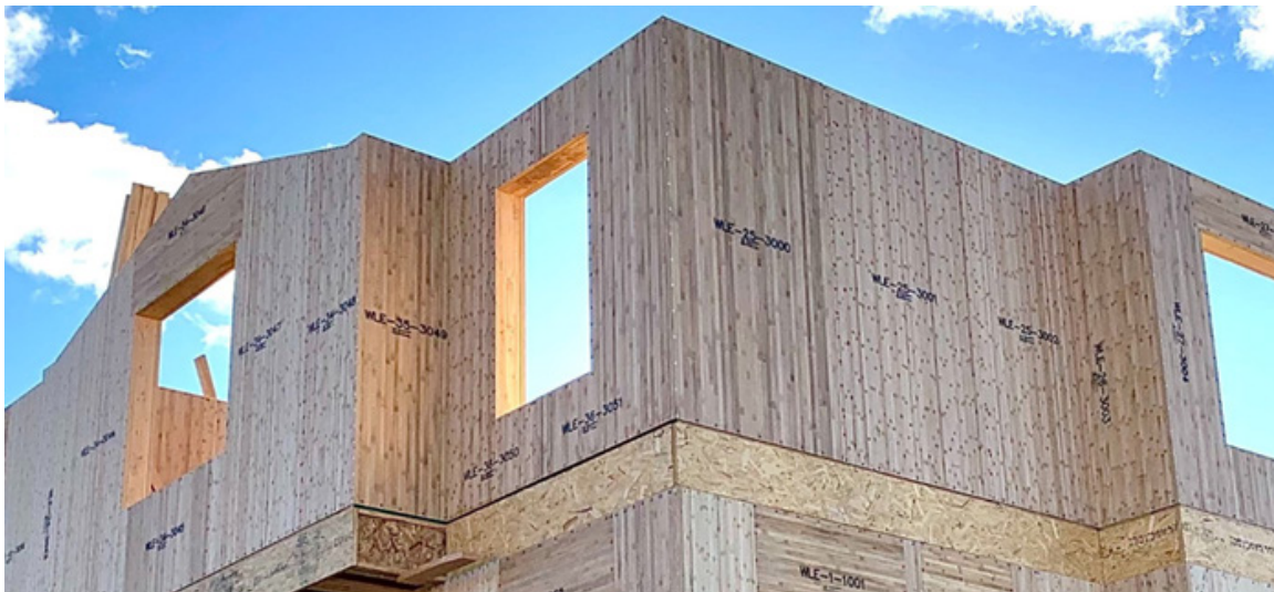
Figure 1. House Under Construction Using BamCore Prime Wall System
